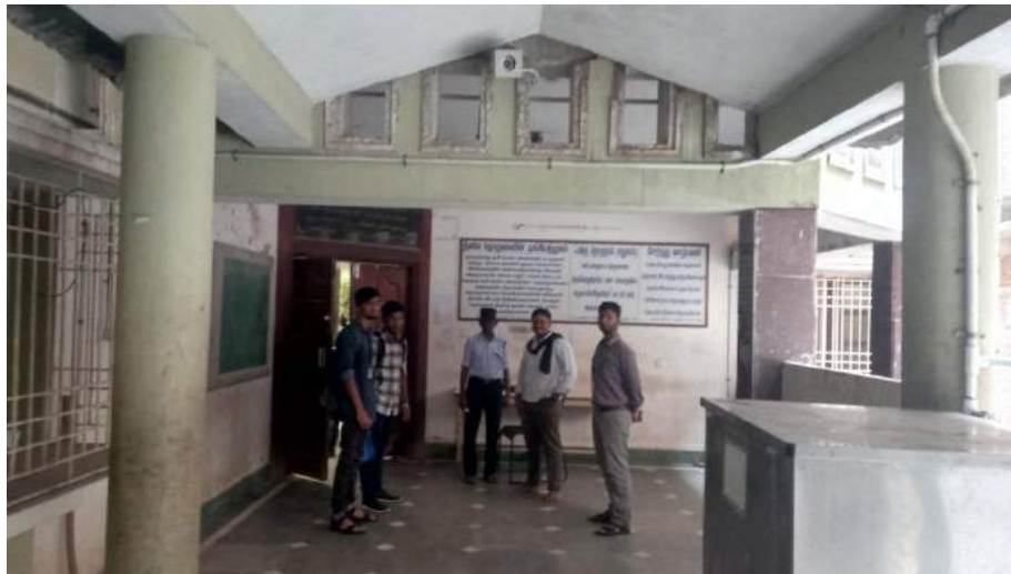
CCTV CAMERA INSIDE THE HOSTEL
